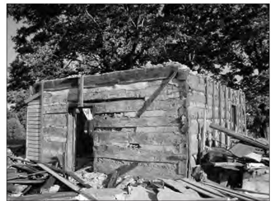
Fig. 19 (below) Henry Ronnebaum's one-room log house, St. Mary's Road, as it is being dismantled in June of 2010. Photograph by Gary Stanton.
