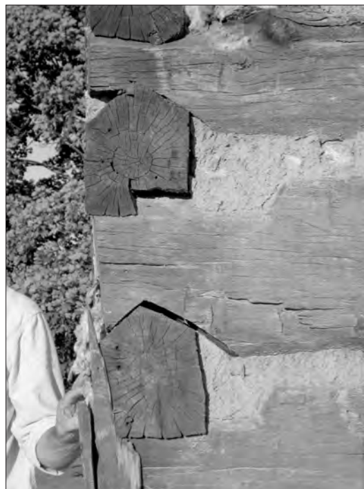
Fig. 21 V-notch corner-timbering on the Ronnebaum house. Photograph by Gary Stanton.
