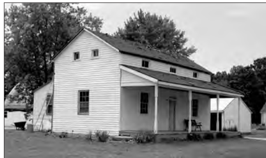
Fig. 28a The Frederick Glaser Family house, ca. 1840, Blue Creek Road, St. Peters, Highland Township. Photograph by Thomas Carter.
