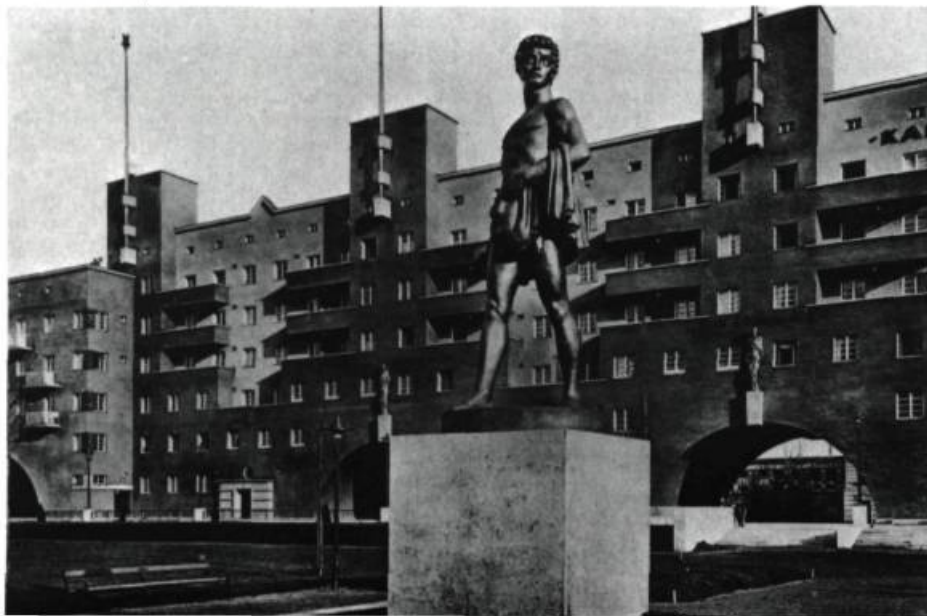
3. Karl EHN, Karl-Marx-Hof (workmen's dwellings), 1927. Main façade.
