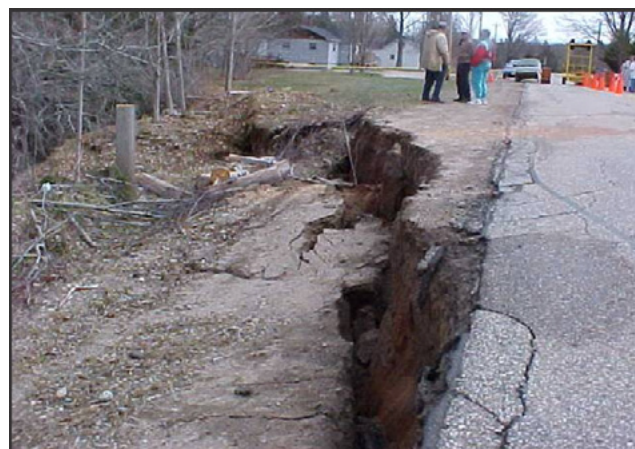
Figure 10. A large rotational slump in Middleton, Nova Scotia. This landslide was associated with fluvial erosion of 20 m-high slope along the Annapolis River when the water table was elevated activating a failure plane between impermeable clay-rich till and overlying outwash sediment.
