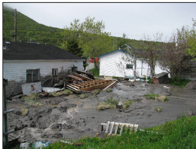
Figure 7. Debris flow deposit at Trout River, Newfoundland. The landslide, though small in volume, detached a house from its foundation and pushed it onto the adjacent road.
