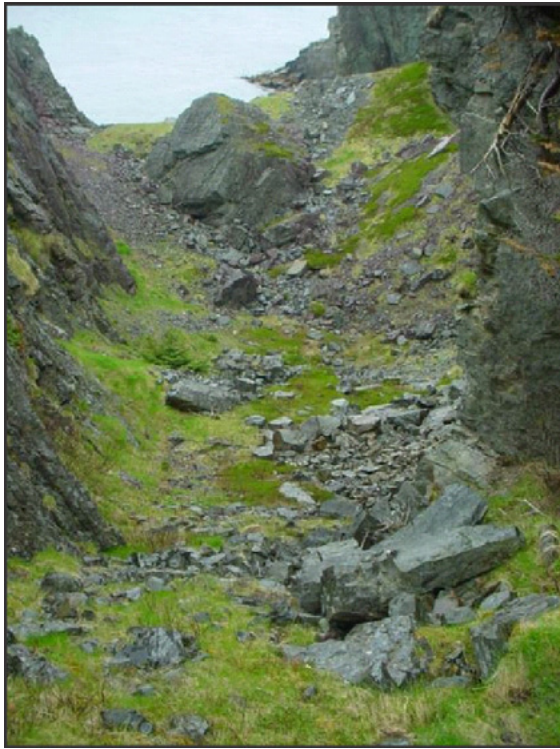
Figure 4. Deadman's Gulch at the entrance to Ferryland Harbour. Before the collapse, the site was believed to have been a sea cave that was frequented to catch baitfish and as a refuge during storms. The large boulder in the background is approximately 10 m across.
