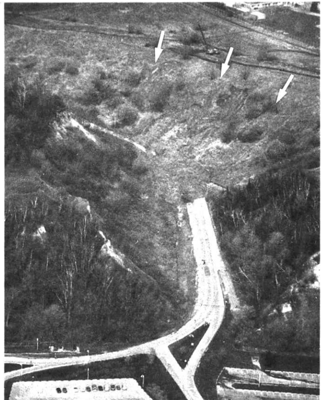
Figure 16 Garbage on the move: recent landslide of April 1991, at Brimley Road along Scarborough Bluffs, involving the downslope failure of municipal waste dumped in a lakeside ravine in the 1950s and 1960s.
