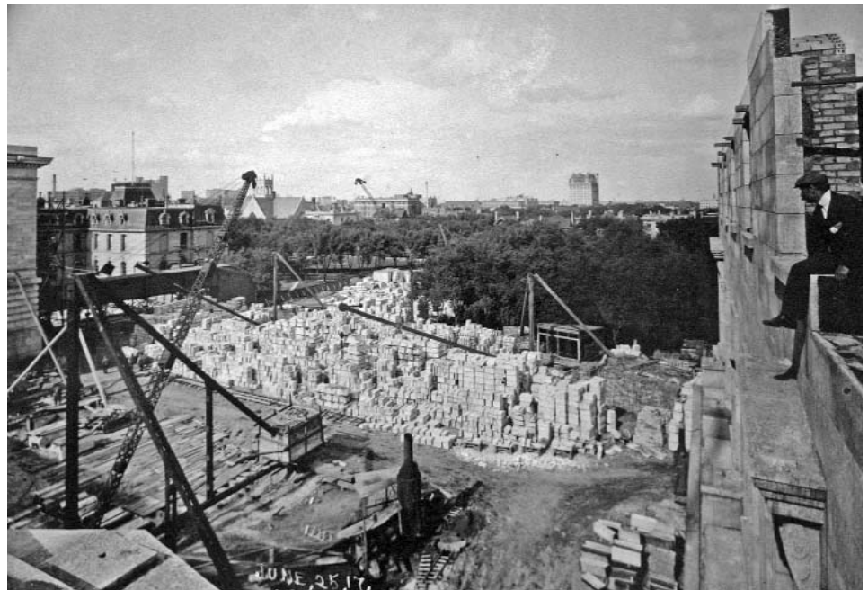
Figure 2. June 1917; an observer on the SE wing of the Legislative Building overlooks the east grounds of the building site (AM, Foote Collection 82). A brick bearing wall with Tyndall Stone facing occurs behind the observer. Blocks of Tyndall Stone are stacked in a staging area below. The old Manitoba parliament building is located on the left side of the photograph adjacent to the NE wing. The Fort Garry Hotel is the tall building in the distance.
