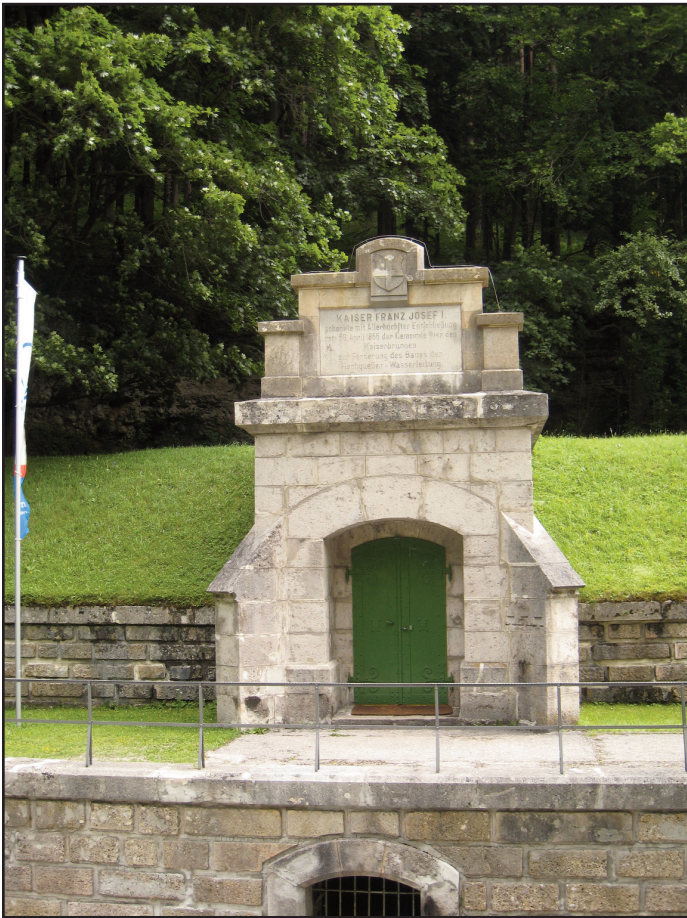
Figure 6b. The waterlock of the Hochquelle at Kaiserbrunnen.
