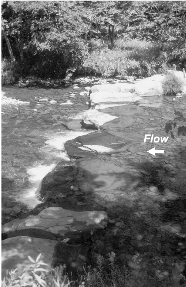
FIGURE 4. Log and rock dam along the Upper Beaverkill River. The support log is hidden under the downstream end of the rock-dam facing. Colonel O'Dell originally constructed this structure in the 1890s.
