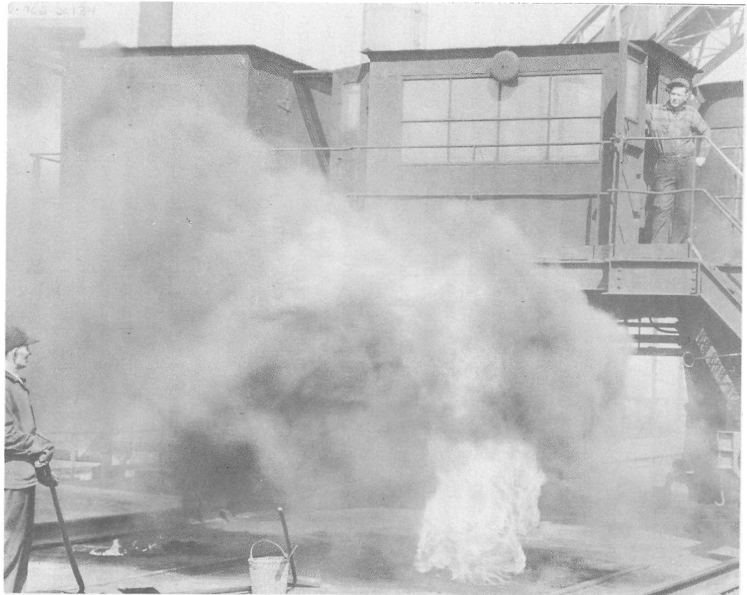
Photograph 2: Coke Ovens. 'You got to open the hole when ... the larry car charges the oven. Got to sweep all the debris into the hold. That's when they make that big puff! Then you have to get the cover back on. They had a little bucket of mud, you just poured it around to seal the hole.'
