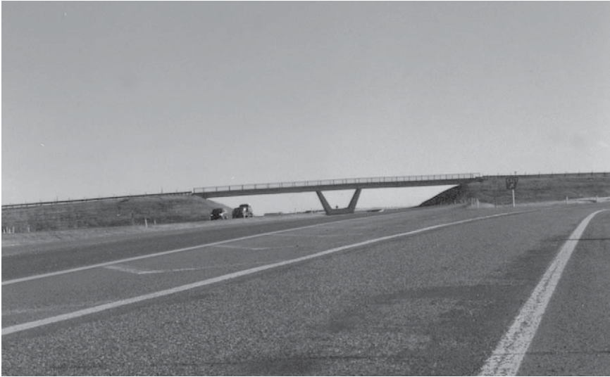
Jumping Pound Grade Separator, Trans-Canada Highway, October 1999.
