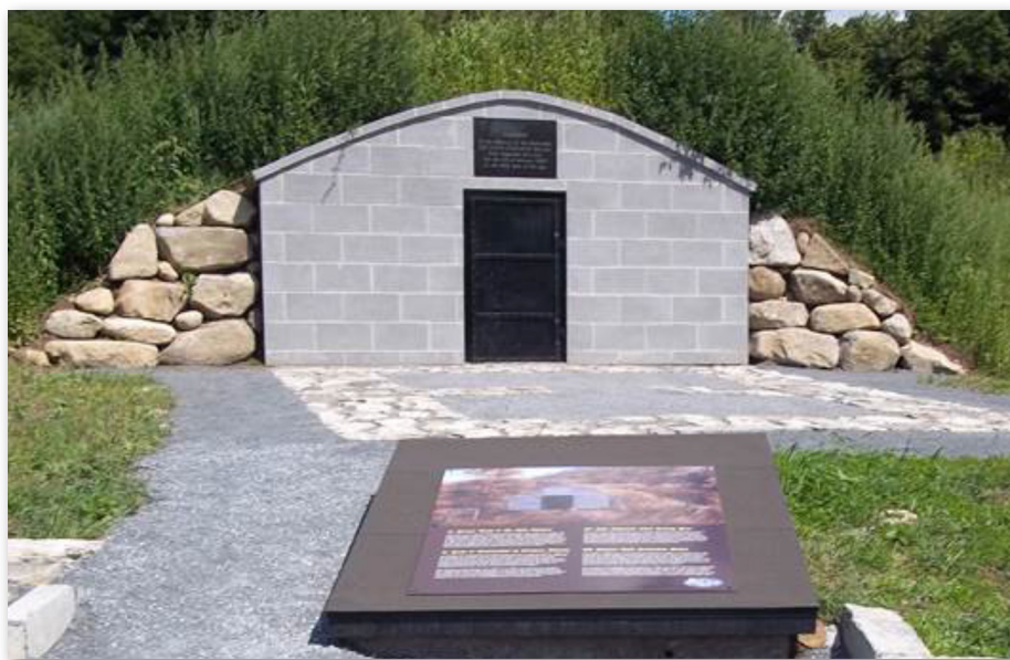
Restored Johnson Family Vault, mont Saint-Grégoire, 2014
