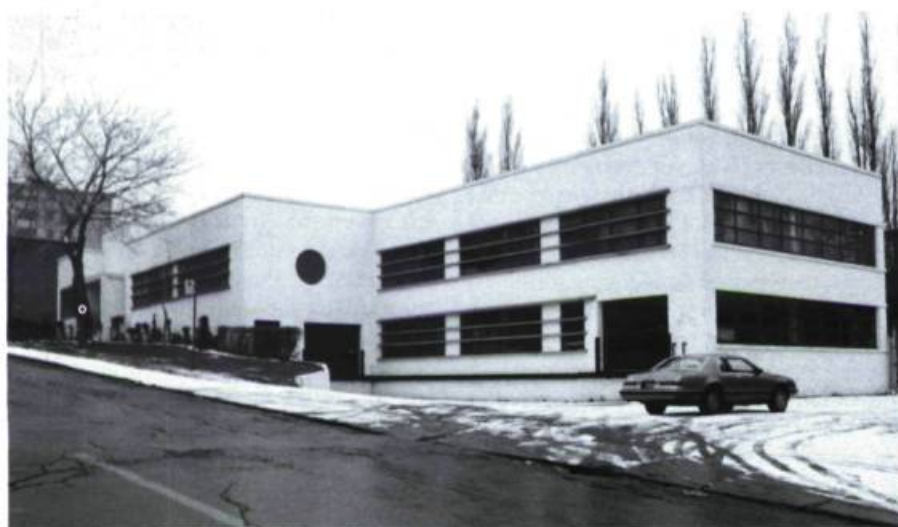
Manufacture Osmose Wood Preserving Co., 1080, Pratt (Perry & Day, arch.; 1945). Photo: P.-R. Bisson et Ass.
