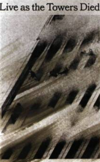
The remains of the World Trade Center's north tower, about a half-mile long, collapsed after the attack on Sept. 11.
