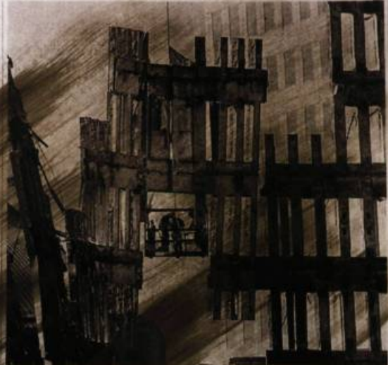
The Final Pieces Welders attached cables to the remaining facade of 2 World Trade Center yesterday in an unsuccessful effort to pull it down. What is left of the building is scheduled to be demolished today.
