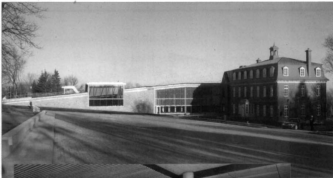
© Croft Pelletier architectes
