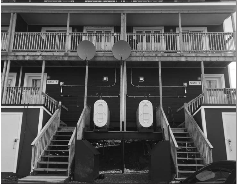
Figure 8. Fuel tanks, storage, stairs and balconies in Iqaluit’s multiplexes contribute to the northern housing vernacular and inadvertently shape the public realm. Image courtesy of author.
