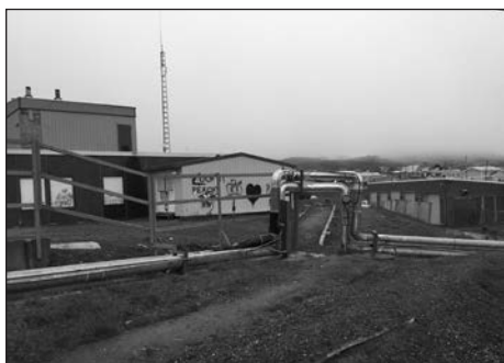
Figures 5. Iqaluit's utilidors appear throughout the city in a haphazard way. In Nuuk, the utilidor is typically paired with the exterior walkways that lead residents to various housing complexes. Images courtesy of author.
