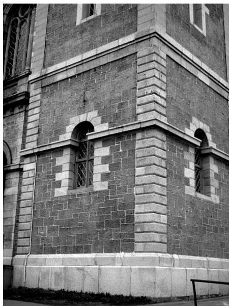
Figure 6 View of the east tower of the Basilica, bases and quoins constructed with Leinster granite and rubble facing with Gilbbett Hill sandstone.
