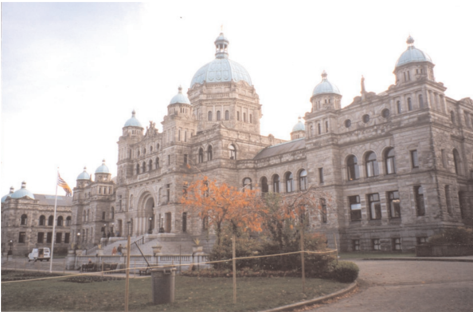
Figure 5. Completed Parliament Building, front elevation looking southeast.
