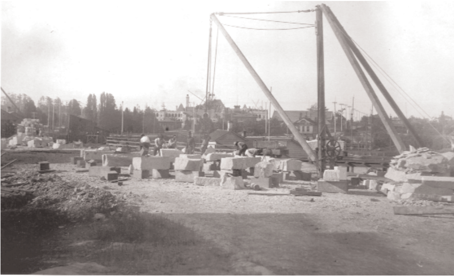
Figure 2. Dressing stone for the British Columbia parliament buildings. British Columbia Archives photo D-02896.
