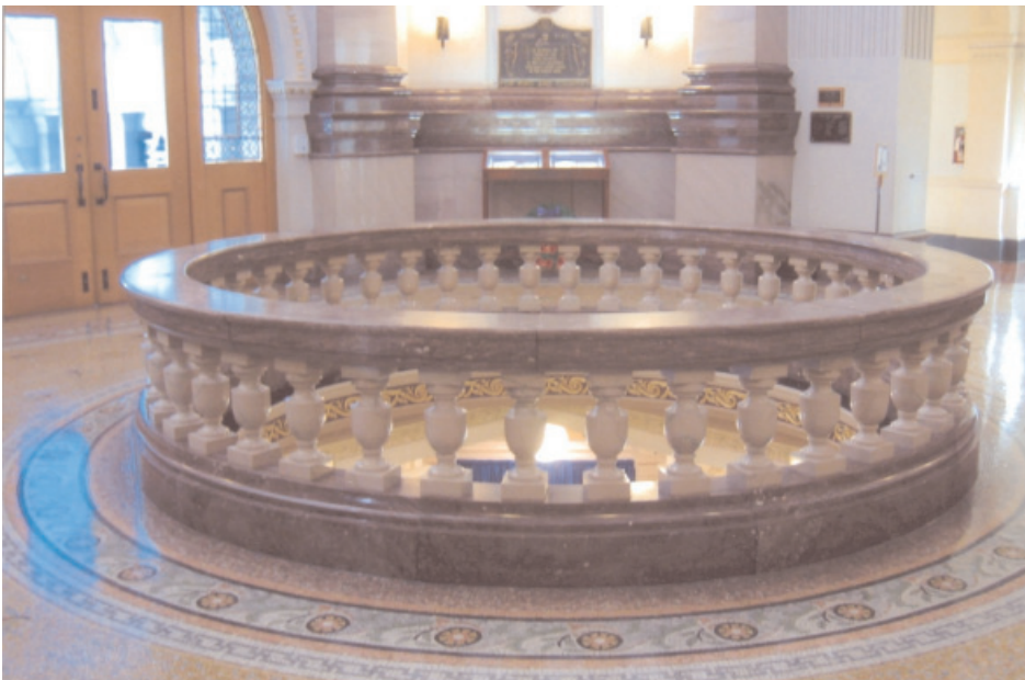
Figure 11. View of the rotunda balustrade.
