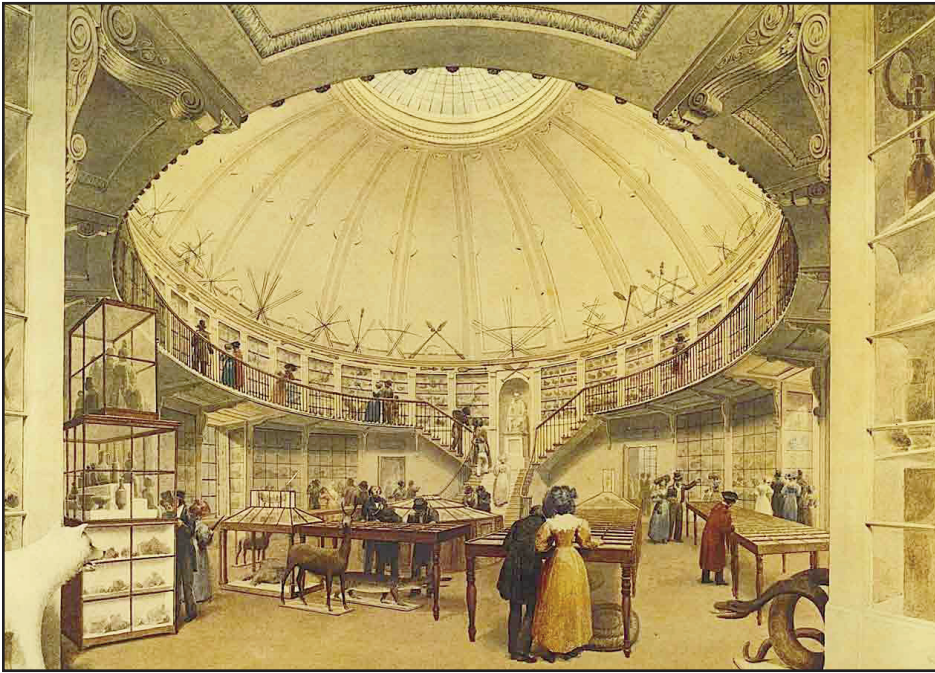
Figure 5. Interior of the Andersonian Museum, designed by James Smith in 1831 as the public face of Anderson's University, now the University of Strathclyde. It was founded in 1796 as an alternative to The University of Glasgow with an emphasis on 'useful learning'. Smith was President of the university in 1831. University of Strathclyde collection.
