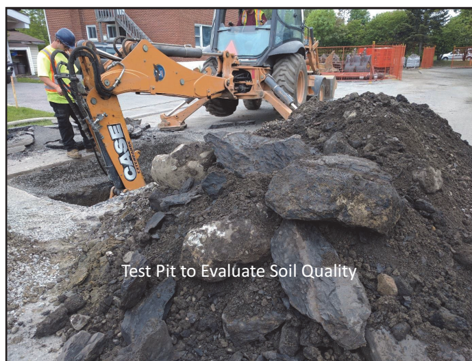
Figure 4. Example of test pit excavation to assess soil quality in the area of infrastructure renewal in Case Study #3.
