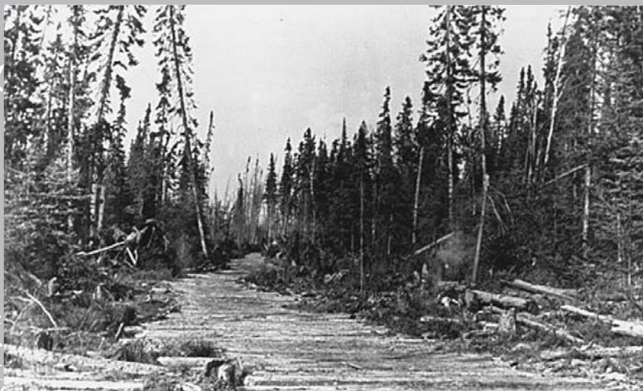
Illustration d'un chemin ponté. (Source : Canadian Heritage Gallery, Corduroy road in Northern Ontario, www.canadianheritage.org/.../transportation0500.htm )
