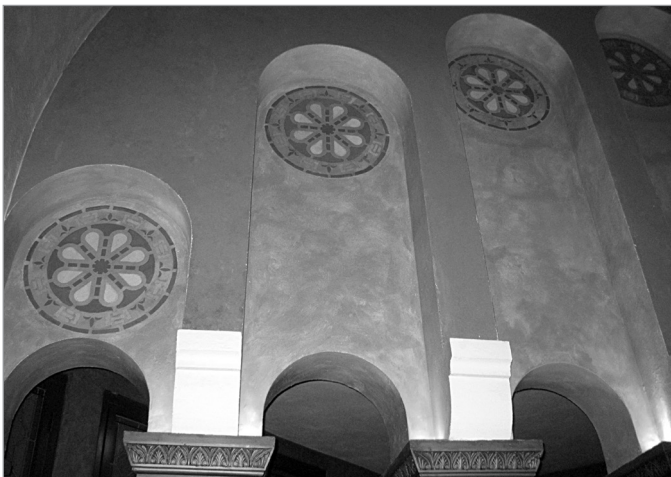
FIG. 11. ORIGINAL STENCIL WORK ABOVE GALLERY ENTRANCES, DOMINION CHALMERS. | NATALIE ANDERSON RATHWELL, 2013.
