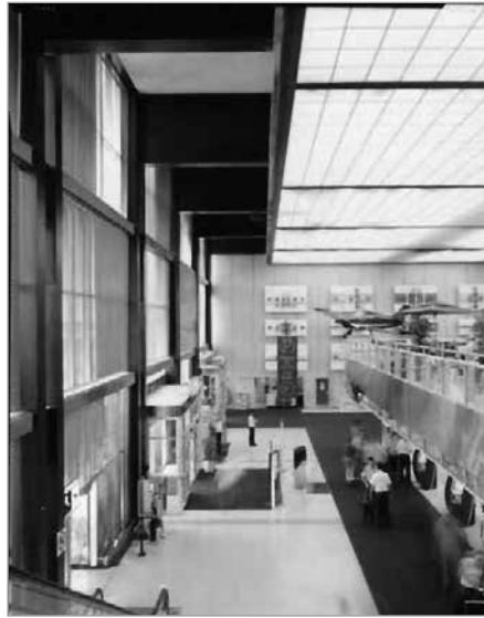
FIG. 6. WINNIPEG INTERNATIONAL AIRPORT 1964. | KESHAVJEE (ED.), WINNIPEG MODERN, P. 88.
