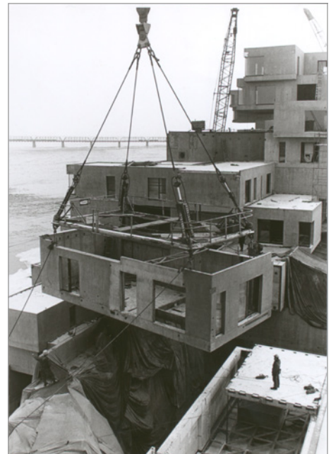
FIG. 19. GANTRY CRANE LIFTING MODULE INTO PLACE, 1966-1967. | SAFDIE ARCHITECTS. SOURCE: MOSHE SAFDIE FONDS, CANADIAN ARCHITECTURE COLLECTION, MCGILL UNIVERSITY LIBRARY, MONTREAL. COURTESY: SAFDIE ARCHITECTS.
