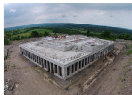
FIG. 19. THE STEEL AND REINFORCED CONCRETE LOWER LEVELS AND PLATFORM OF THE MAIN DHARMA HALL AT THE WUTAI SHAN BUDDHIST GARDEN, 708 SKI HILL ROAD, BETHANY, ON. | BUDDHIST ASSOCIATION OF CANADA'S CHAM SHAN TEMPLE: [HTTP://THEBUDDHISTGARDEN.COM/GALLERY%E7%9B%B8%E7%89%87%E9%9B%86/MAIN-HALL-CONCRETE-FOUNDATION%E5%A4%A7%E6%AE%BF%E6%B0%B4%E6%B3%A5%E5%9F%BA%E7%A4%8E%E5%BB%BA%E8%A8%AD/], ACCESSED APRIL 5, 2021.
