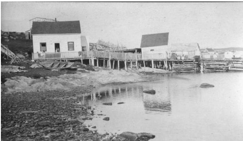
Figure 6. Photograph 1.01.114. Hancock House.
