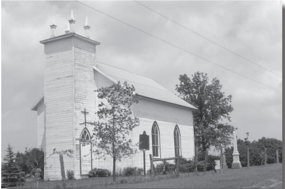
FIGURE 6. St Mary's Anglican church faces east on the north side of a country road. The overhead wires show the road alignment, and the entrance is positioned towards it. Metcalfe Township Road 5, Middlesex County, 1979.
