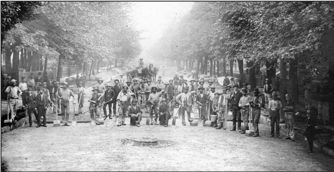
Paving Streets and lining pockets – a work crew pauses for a photo opportunity on Jarvis Street. City of Toronto Archives Fonds 200 Former City of Toronto fonds. –1834-1997, Series 376 City Engineer’s Dept. photographs. – 1891-1911, File 1, Item 22
