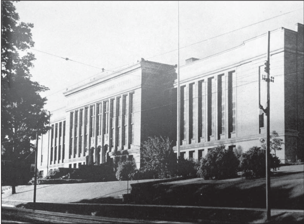
Figure 1: Photo of K.C.I. from the Grumbler , 1945-1946.
