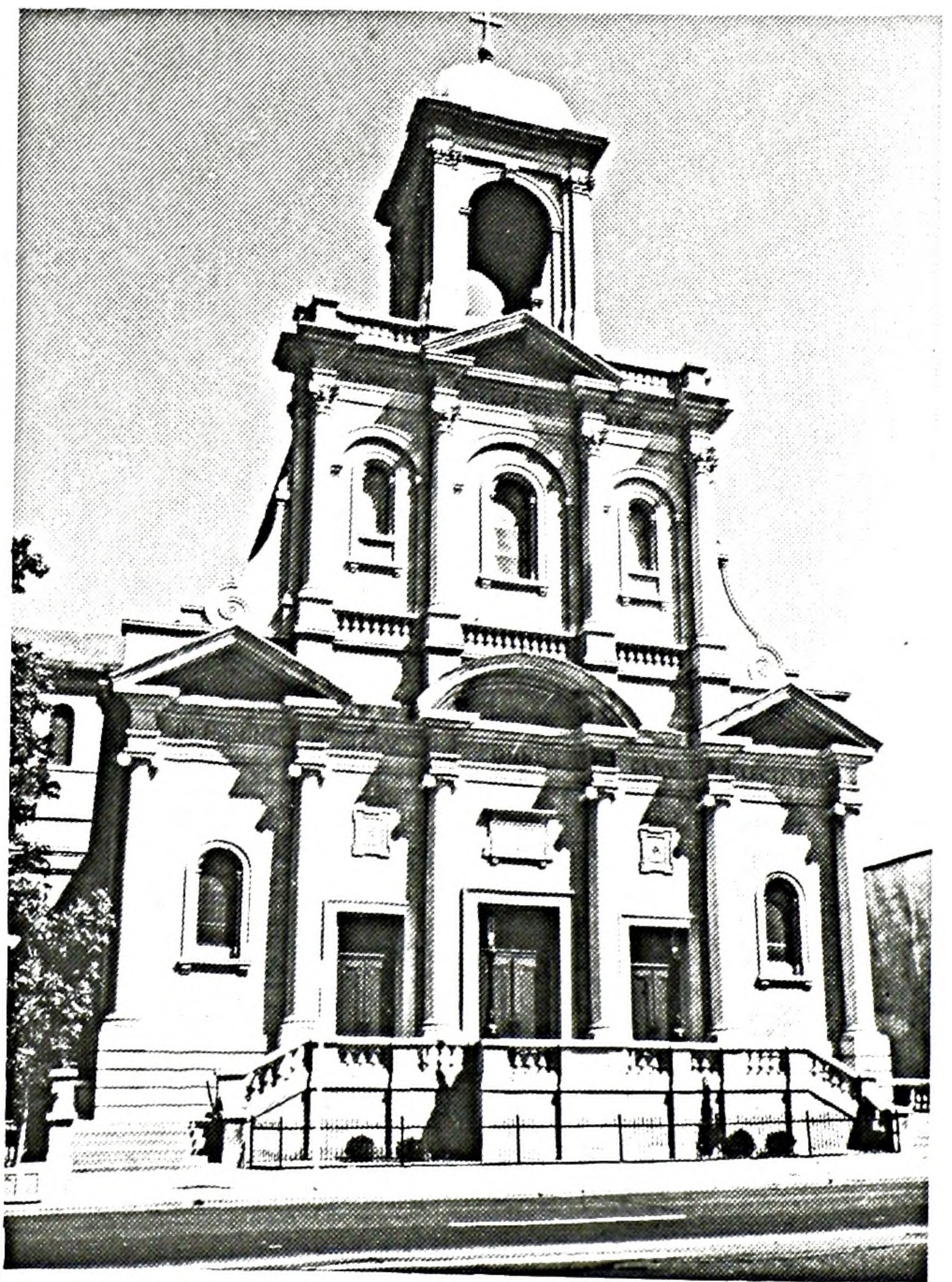
FIGURE 26. A.W. Holmes, Holy Name Church, Toronto, basement 1914-15, upper church dedicated 1926. Main façade (Photo: M. Thurlby).
