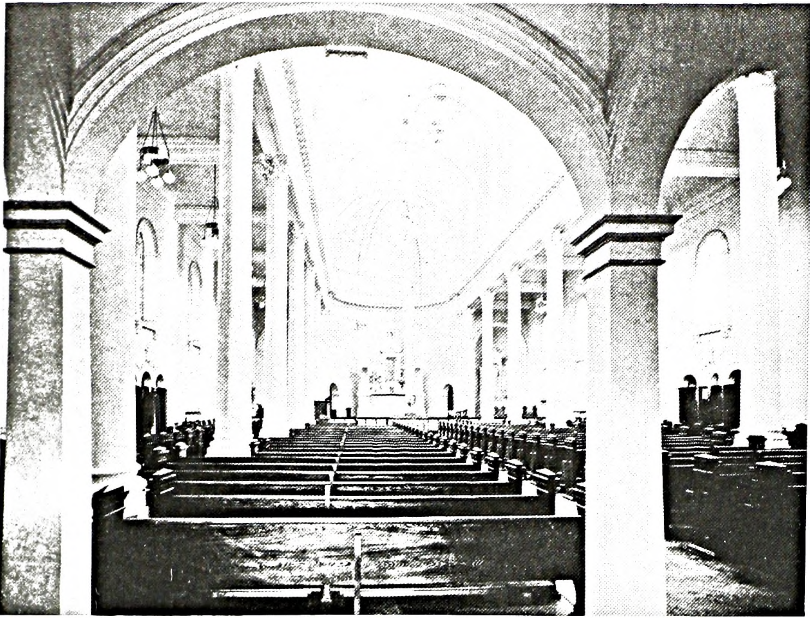
FIGURE 25. St. Ann's Church, Toronto. Interior looking east, after Construction , VIII (December 1915), p. 497 (Photo: Metro Toronto Library Board).
