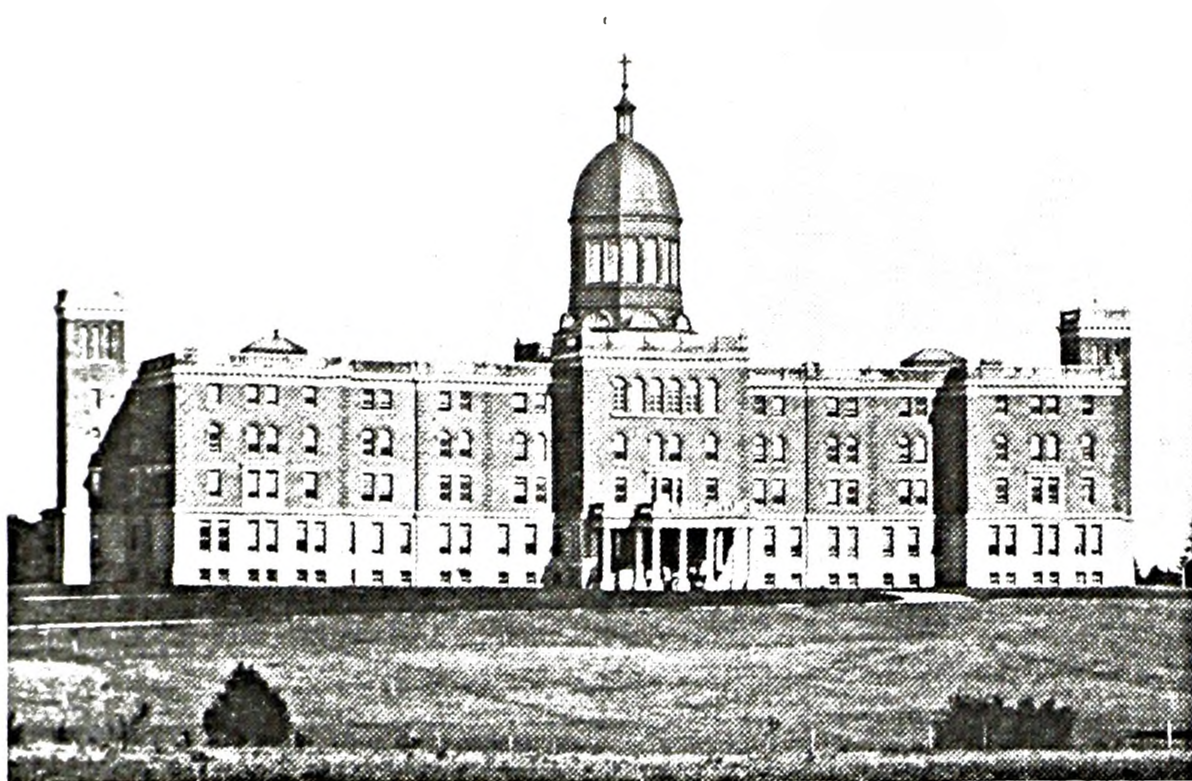
FIGURE 21. St. Augustine's Seminary. General view from the west, after Construction , VIII (December 1915), p. 486 (Photo: Metro Toronto Library Board).
