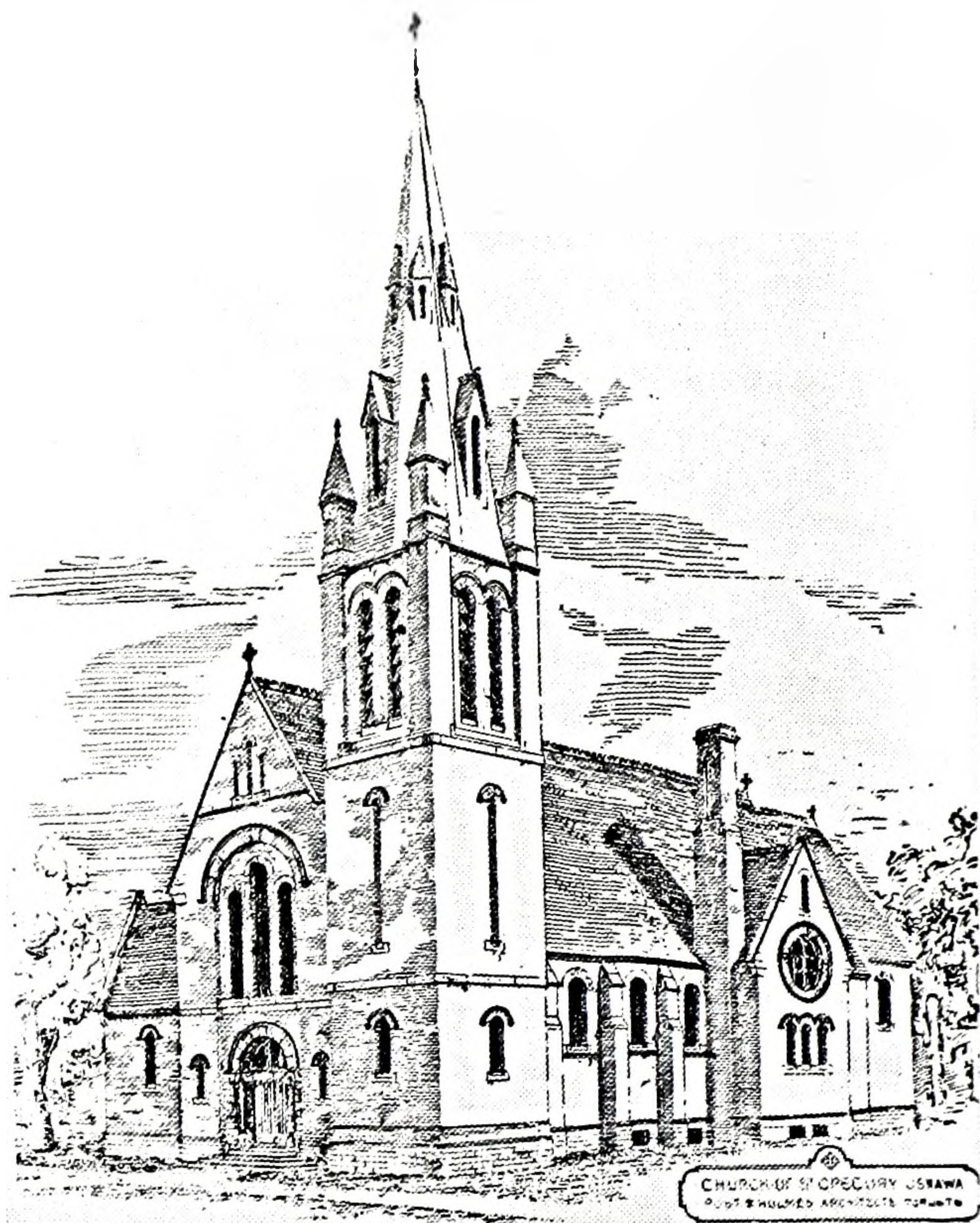
FIGURE 13. Post & Holmes, St. Gregory's Church, Oshawa, 1894-5. After CAB , viii (February 1895), illustrated supplement (Photo: Metro Toronto Library Board).
