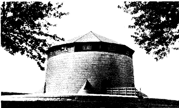
MURNEY TOWER, MACDONALD PARK, KINGSTON, ONTARIO.
