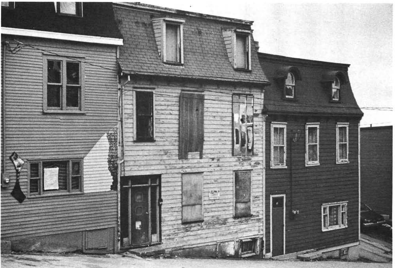
A dilapidated, vacant house on Victoria Street.
