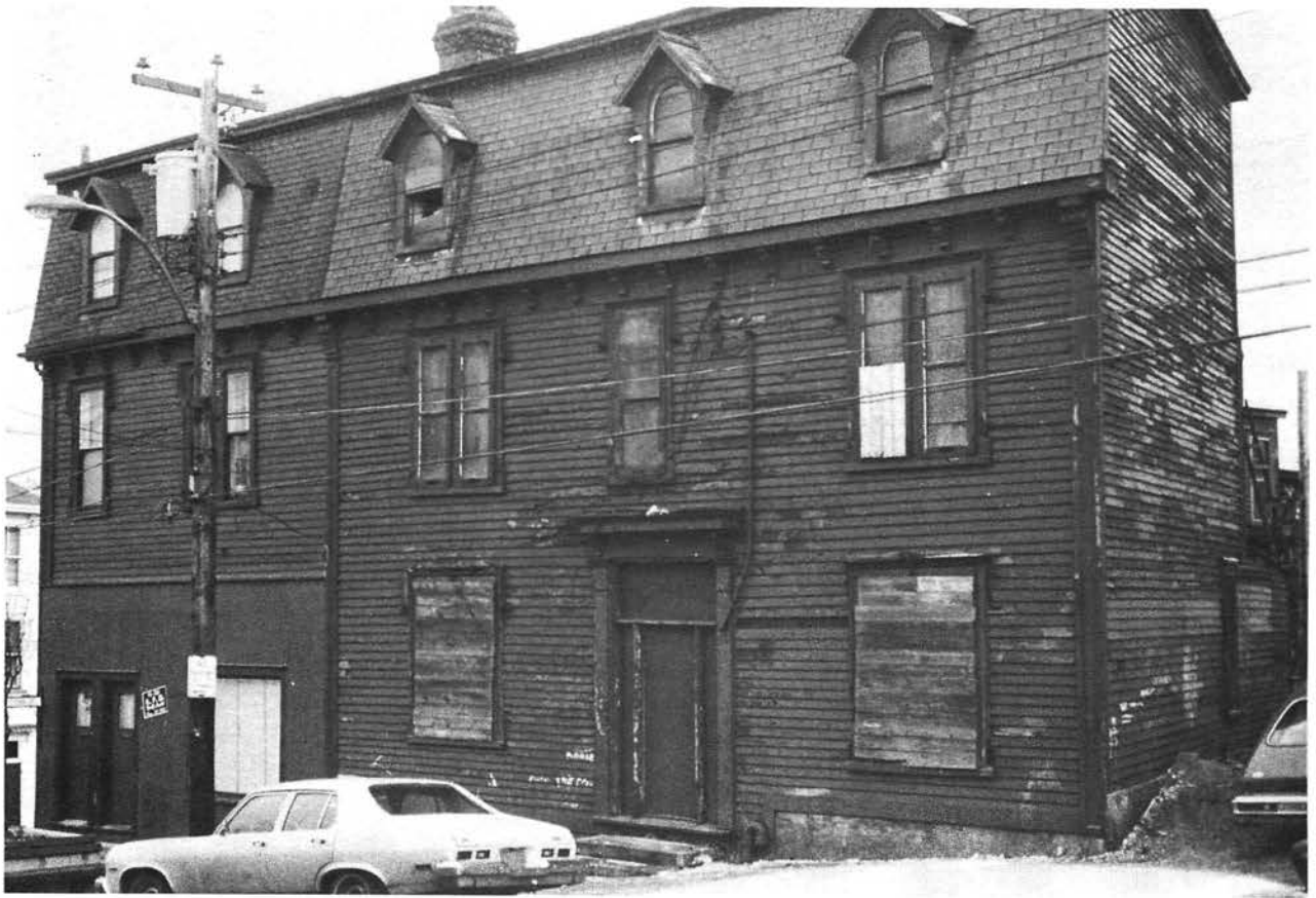
An abandoned house on Gower Street.
