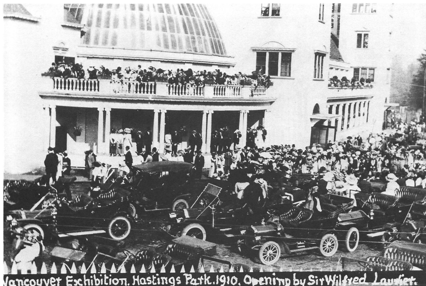
FIGURE 6. Opening of the Vancouver Exhibition Building in Hastings Park by Sir Wilfrid Laurier, August 16, 1910. Photographer unknown.
