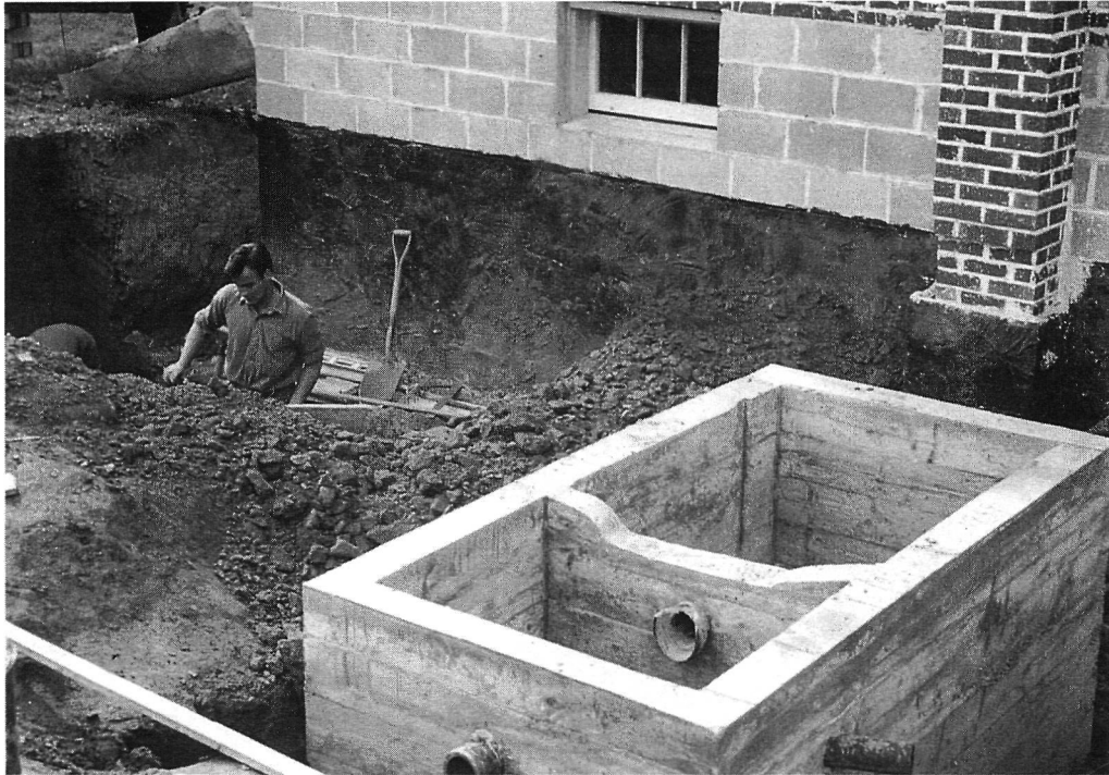
Figure 14: The septic tank was poured, and Harry Hall prepared to frame in the cistern, September 1949.
