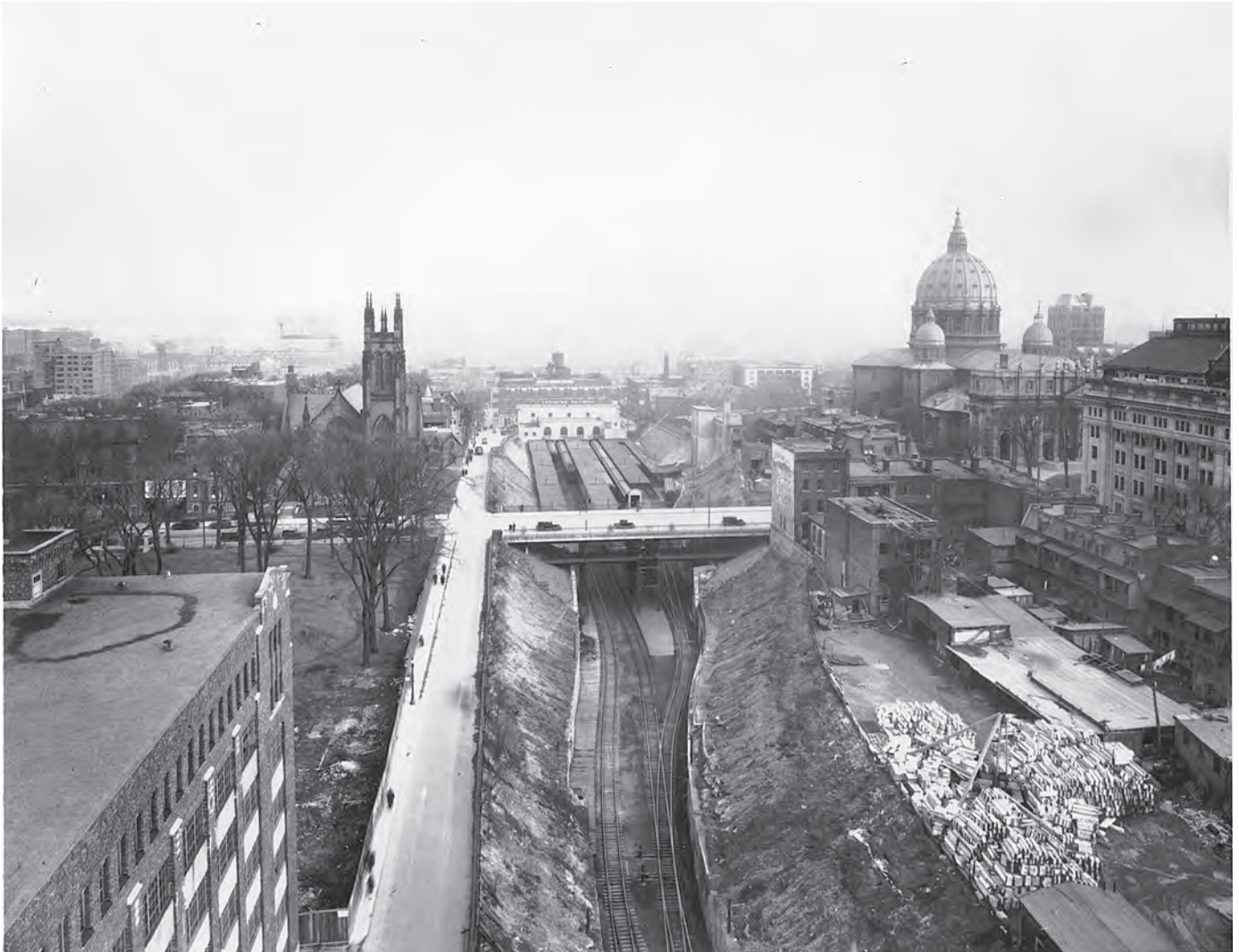
Figure 1: Looking south, Canadian National Railway pit, near Dorchester Street, Montreal, 1930 (McCord Museum MP-1989.20.2).
