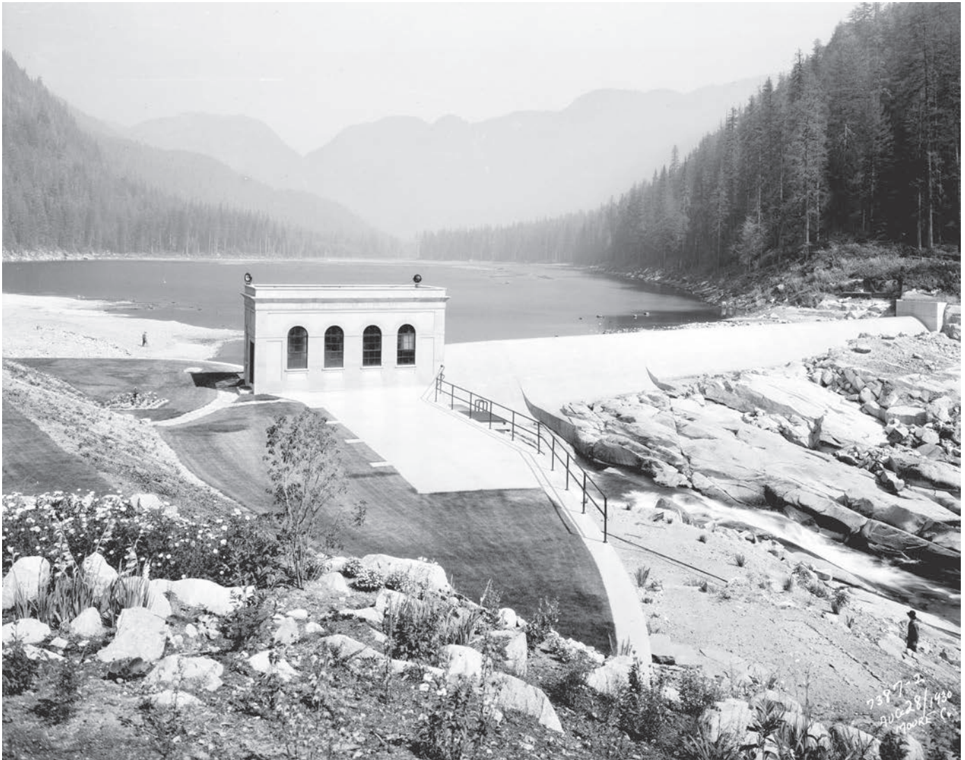
Figure 3: The dam at Seymour Falls was completed in 1926 and was crucial to transforming the river from being a natural waterbody with seasonal highs and lows into a reservoir tank that could be controlled to supply Vancouver with water. The building contained the screen house, through which the water passed before it was sent through a 60-inch, wooden conduit roughly four miles down the mountain to the city's distribution mains. The local grounds were also landscaped to improve their aesthetic appeal. Source: City of Vancouver Archives, mount N38.2, photographer W.J. Moore.
