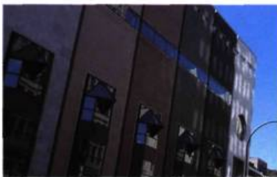
Façade, rue Crescent (2) .
