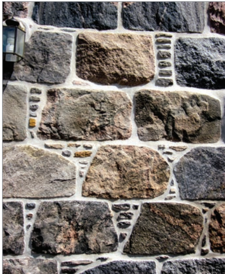
FIG. 15. PINNINGS FILLING GAPS BETWEEN STONE BLOCKS BY AN ANONYMOUS CRAFTSMAN, 35 TH LINE, NO 6432, NEAR EMBRO, OXFORD COUNTY. | KAREN E. ARMSTRONG.
