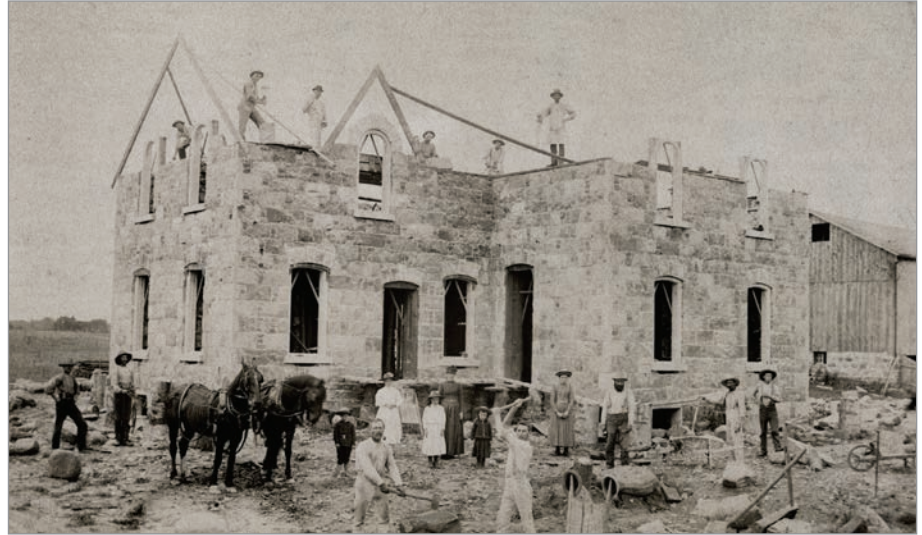
FIG. 22. LAWRENCE HOUSE, CONSTRUCTION SITE, 1891, 205 ALLEN ST., THAMESFORD, OXFORD COUNTY. | AMERICAN AGRICULTURIST , 1894, SPECIAL THANKS TO LISA BICUM AND GEOFF ELLIS.
