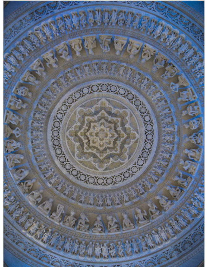
FIG. 13. CEILING OF CORBEL CONSTRUCTION USED TO TRANSITION FROM A SQUARE TO A CIRCLE. | BAPS TORONTO. COPYRIGHT HELD BY BAPS SWAMINARAYAN SANSTHA.
