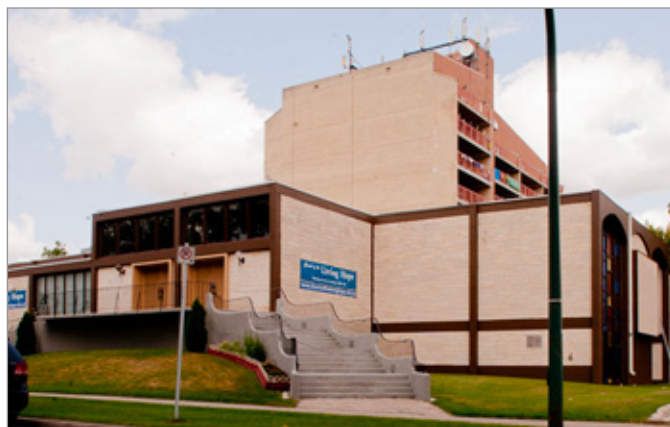
FIG. 10. EXTERIOR OF B'NAY ABRAHAM SYNAGOGUE. | WINNIPEGARCHITECTURE.CA, [HTTPS://WWW.WINNIPEGARCHITECTURE.CA/235-ENNISKILLEN/], ACCESSED MARCH 11, 2021.
