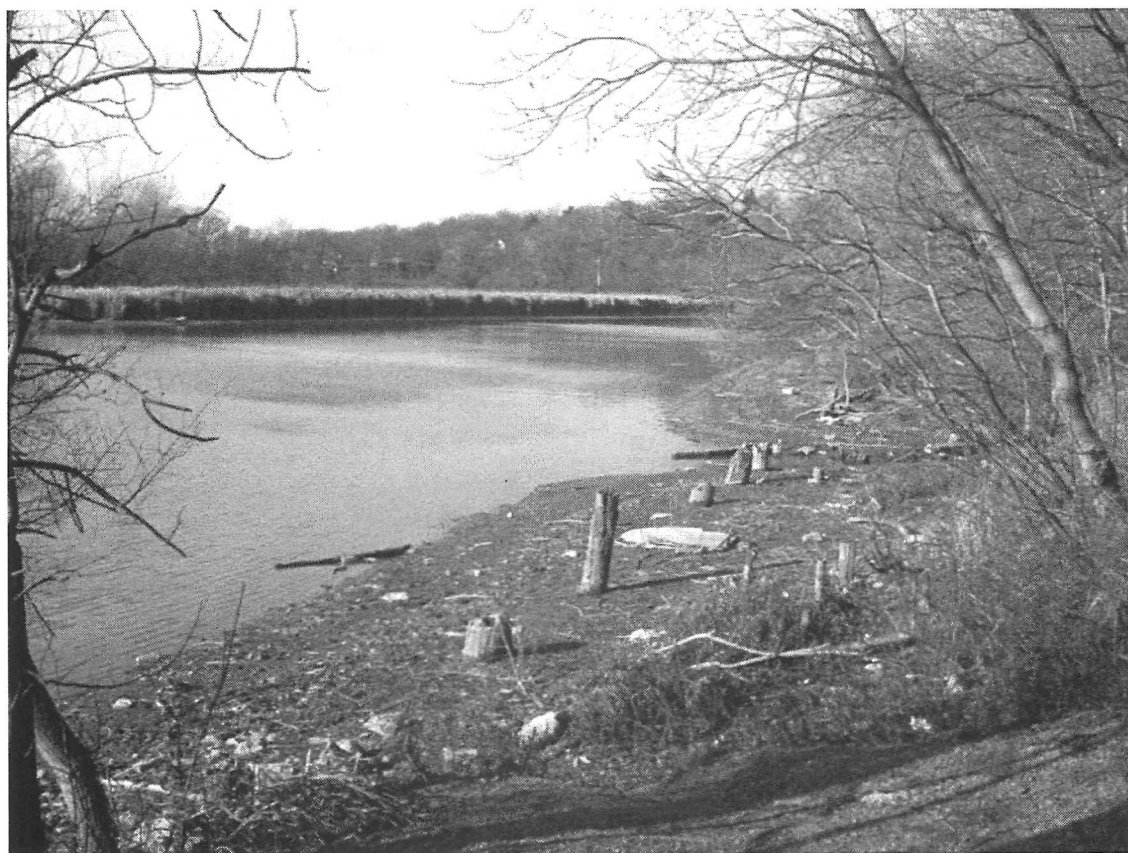
Figure 5 Rotted posts of the old pier. Photo: Diane Boyer
