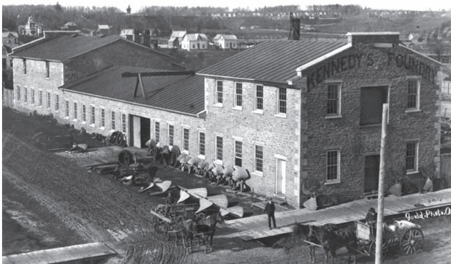
William Kennedy & Sons Co. Foundry at the corner of Stephens St. and Beech St. (now 1 st Ave. West and 11 th St. West). Notice the wooden patterns located along side the building. Also of note is the wooden boardwalk used as a sidewalk. This photograph dates c.1900. The Grey Roots Archival Collection, 1973.010.019
