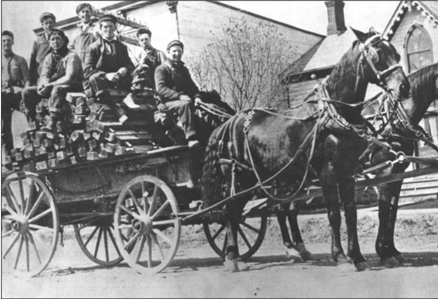
Linesman taking a wagon of crossarms to repair telephone lines. 989.21.3
