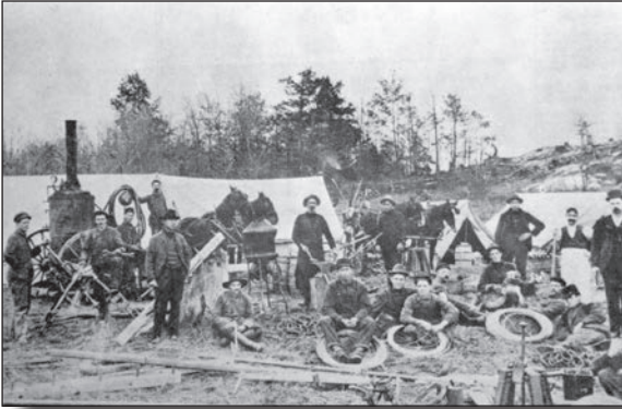
The construction of the line connecting Owen Sound to Meaford, 1886, 990.5.12
