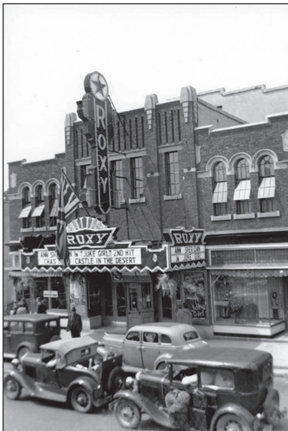
The Roxy theatre, 1942. Unknown source. < https://www.reddit.com/r/barrie/comments/3qqcdu/roxy_theatre_dunlop_st_w_1942/ >
