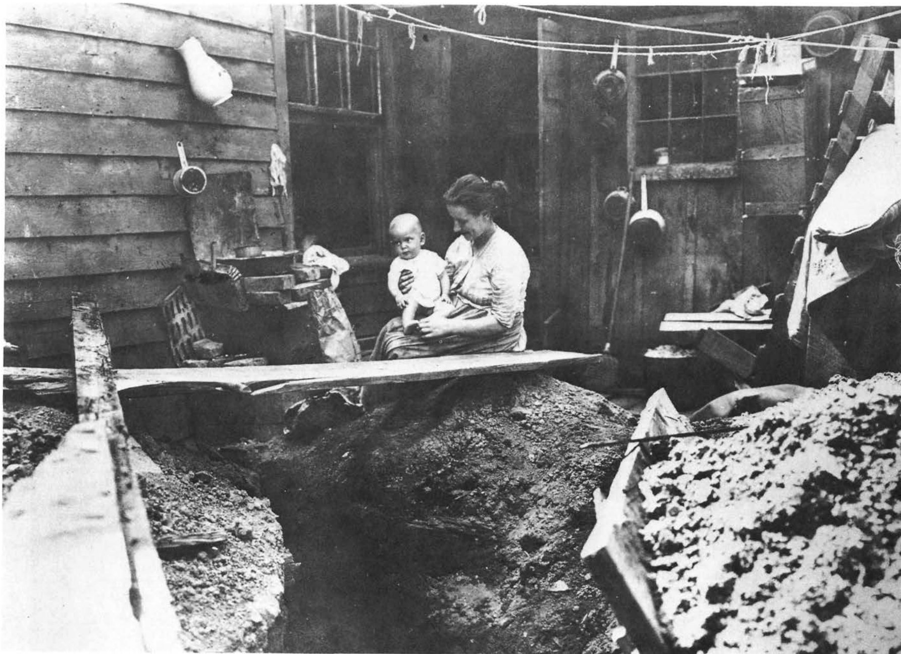
Summer 1912. Rear of #94 Elizabeth Street. Drain being installed to connect with Chesnut Street Sewer. James Collection - City of Toronto Archives
