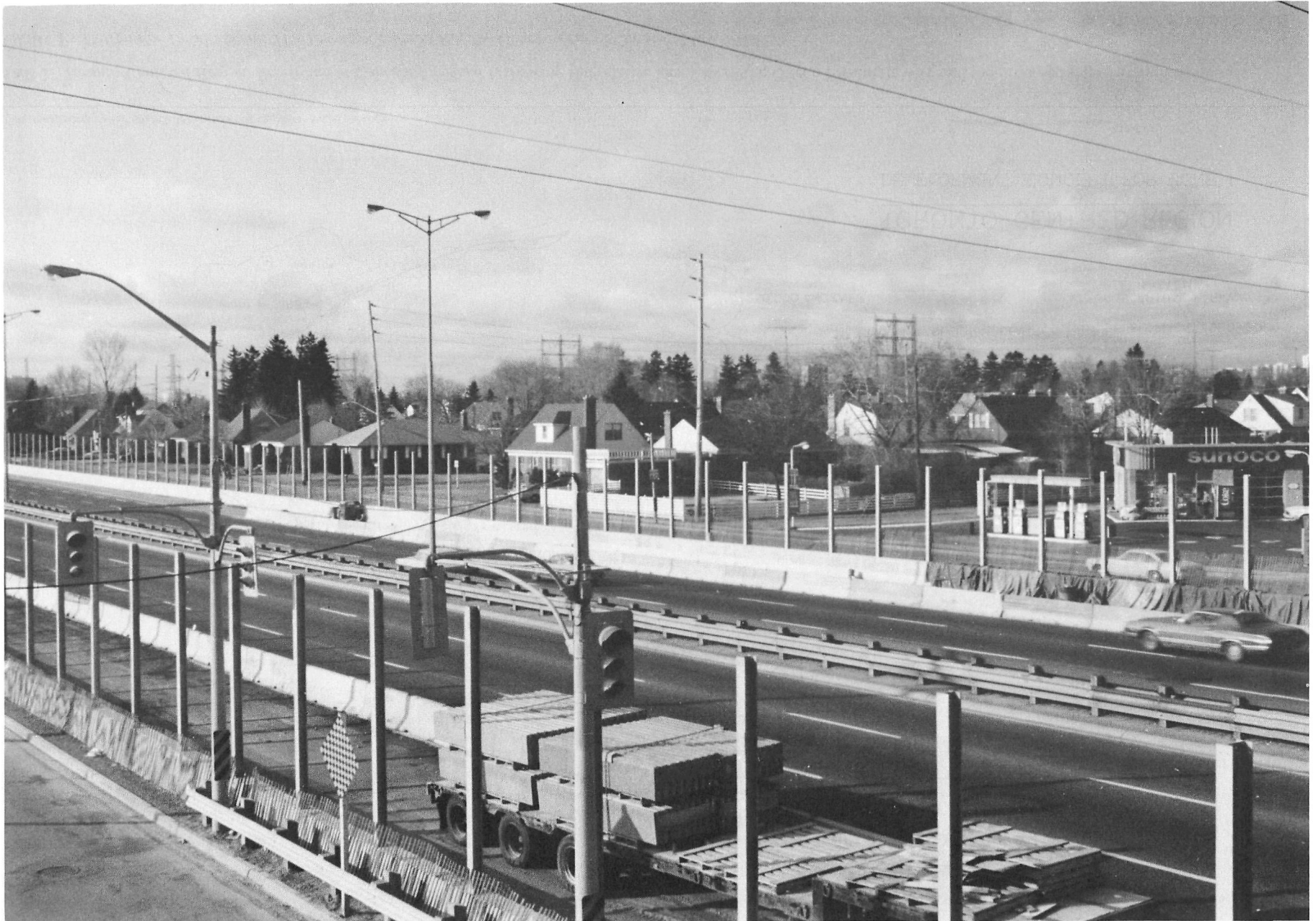
FIGURE 12. Erecting “noise-barriers” along the Queen Elizabeth Way, west of Dixie Road, 1983.
