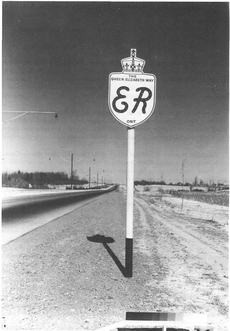
FIGURE 1. A new signpost erected along the Queen Elizabeth Way near Bronte. At this time, double lighting fixtures were located within the central median.
