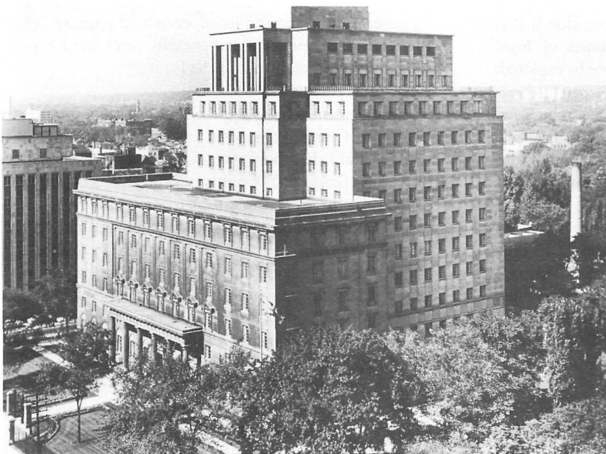
c) Head Office Building of 1924-25 (left) and Head Office Addition 1949-52 (right), photo c. 1955.
