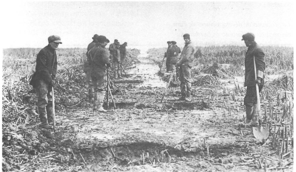
Photo 1: Reclamation Work in Progress, Ashbridge's Bay, 21 November 1914
