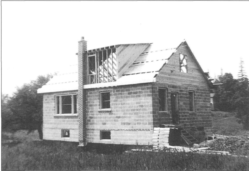
Figure 13: The house as it approached completion in late summer 1949. Owner-builders like the Halls favoured concrete blocks since they were comparatively cheap and easy to lay.
