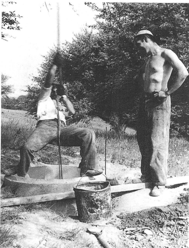
Figure 9: Harry Hall (left) and Bill Cameron (right) digging the first well, that eventually collapsed, June 1949.
