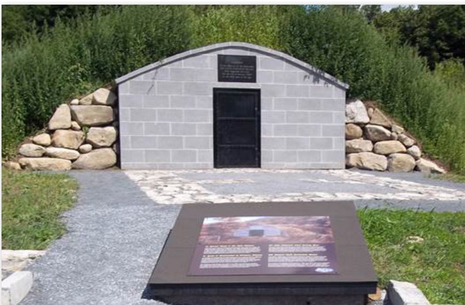
Restored Johnson Family Vault, mont Saint-Grégoire, 2014
