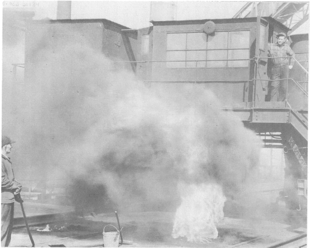
Photograph 2: Coke Ovens. 'You got to open the hole when ... the larry car charges the oven. Got to sweep all the debris into the hold. That's when they make that big puff! Then you have to get the cover back on. They had a little bucket of mud, you just poured it around to seal the hole.'
