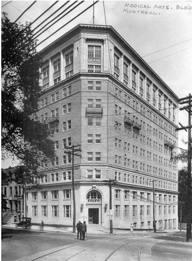
Figure 2. Montreal Medical Arts Building.
